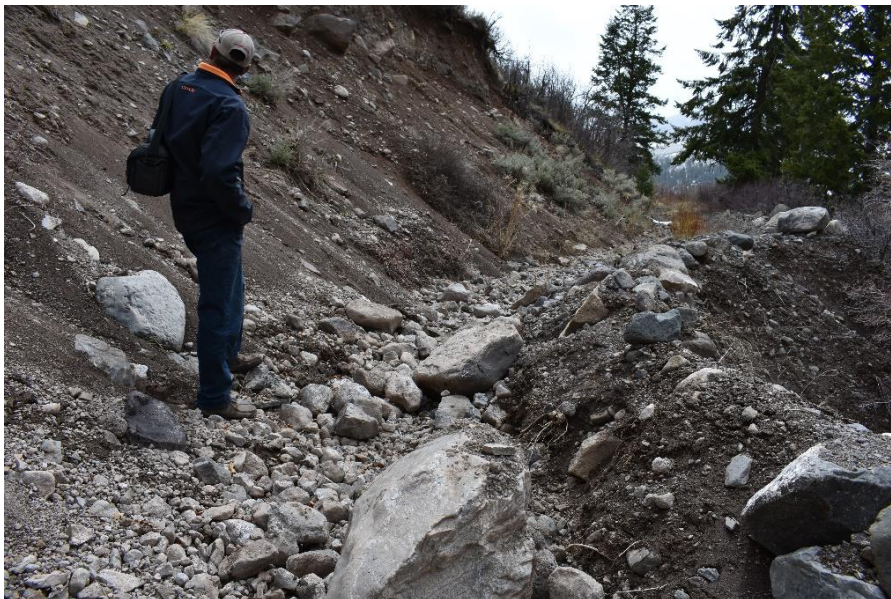
Irrigation ditch in slide area. Piping damage-prone sections of open ditches improves the reliability of water delivery and reduces maintenance.
