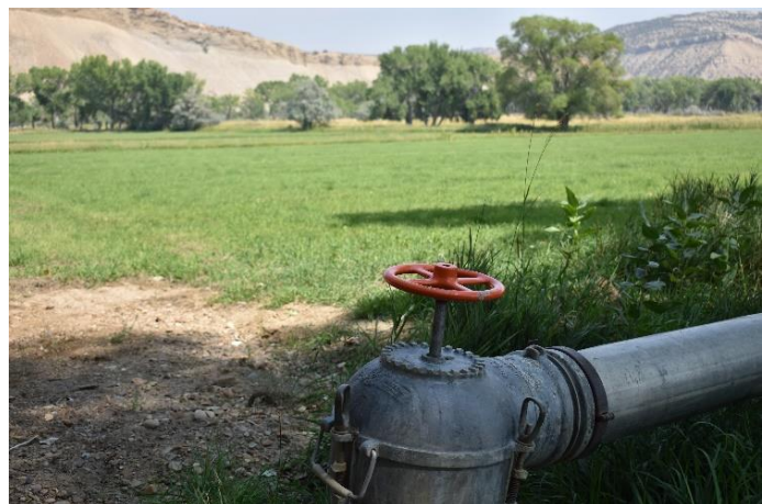
Valve and irrigation pipe. Photo: Phil Brink
