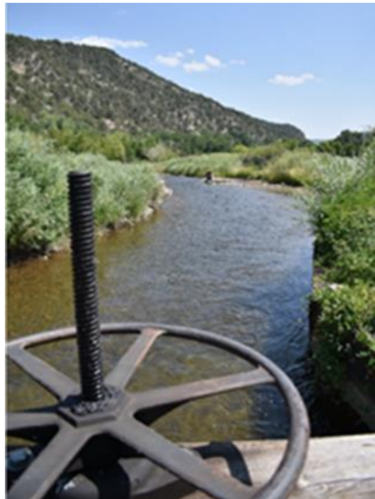
Diversion channel and headgate. Photo: Phil Brink
