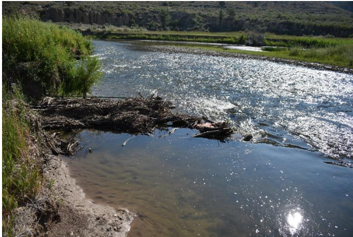
Diversion structure damaged by high flows and debris. Photo: Phil Brink
